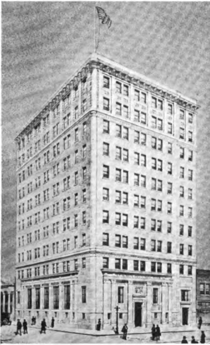
Ouachita National Bank, Monroe, La., a bank building in one of our smaller cities that in the beauty of its architecture equals the best structure in any community. It is now being built by the Underwood Contracting Corporation.
