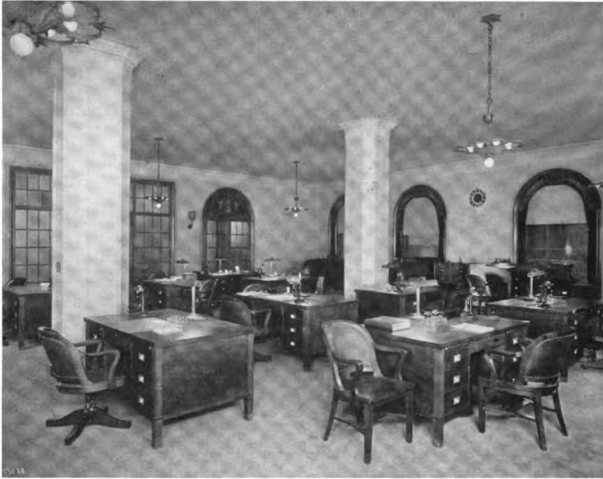
Officers' Quarters. Showing Entrance to Directors' Room
