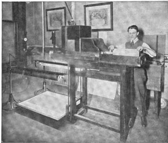
This Cut Shows a Photostat Installation
