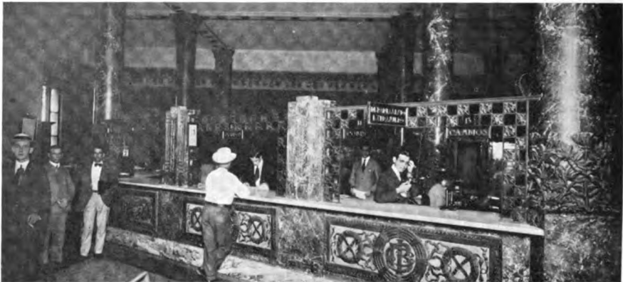
Another View of the Lobby Banco Internacional de Cuba
