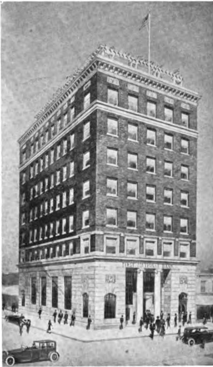
This new building for the First National Bank, Crowley, La., is now being erected by the Underwood Contracting Corporation. It will be Crowley's first skyscraper
