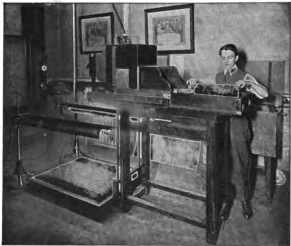
This Cut Shows a Photostat Installation
