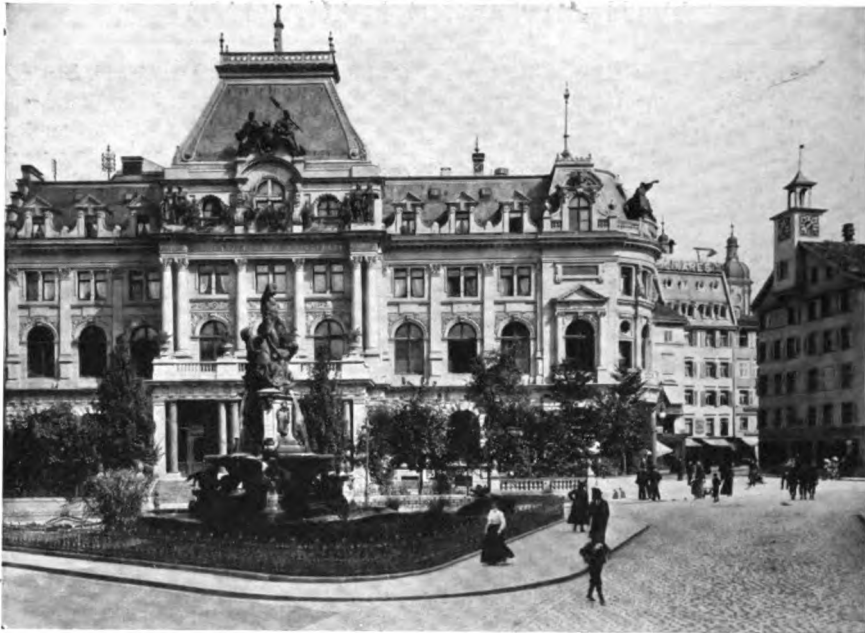
St. Gall Office Swiss Bank Corporation
