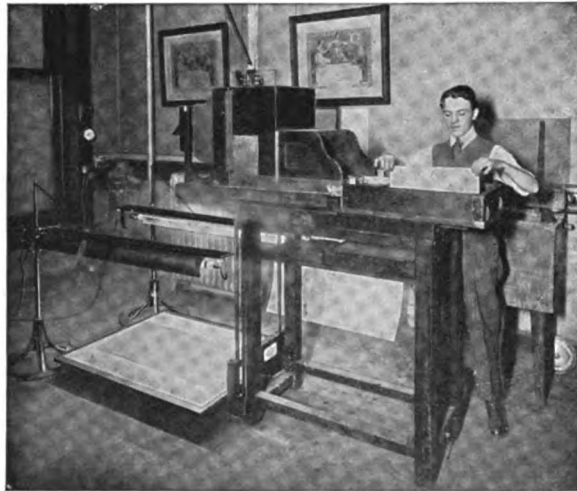
This Cut Shows a Photostat Installation
