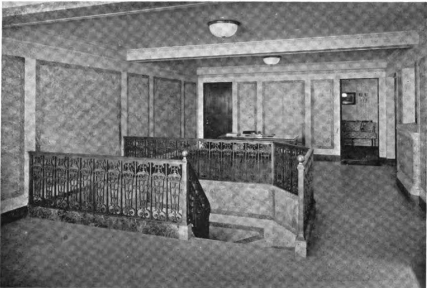
Stairway Leading to Safe Deposit Vaults, National American Bank of New York
