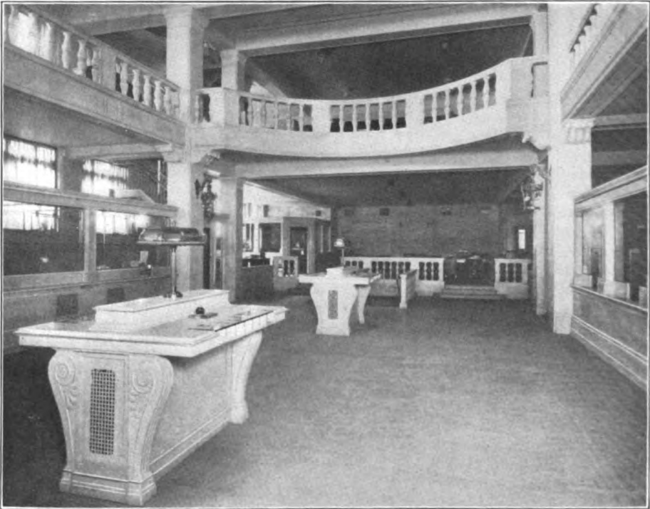
Main Lobby, Officers Quarters in Rear
