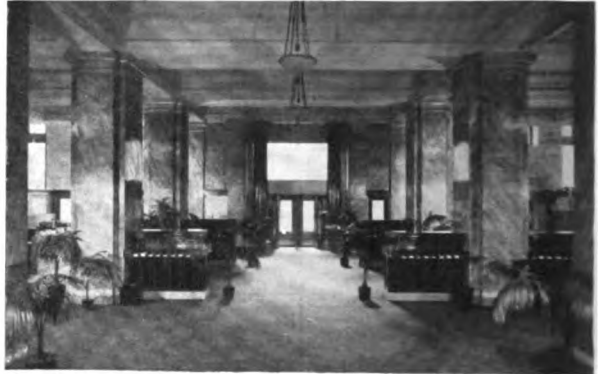
Main corridor, looking toward main entrance
