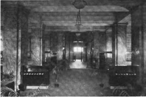
Main corridor, looking toward rear entrance
