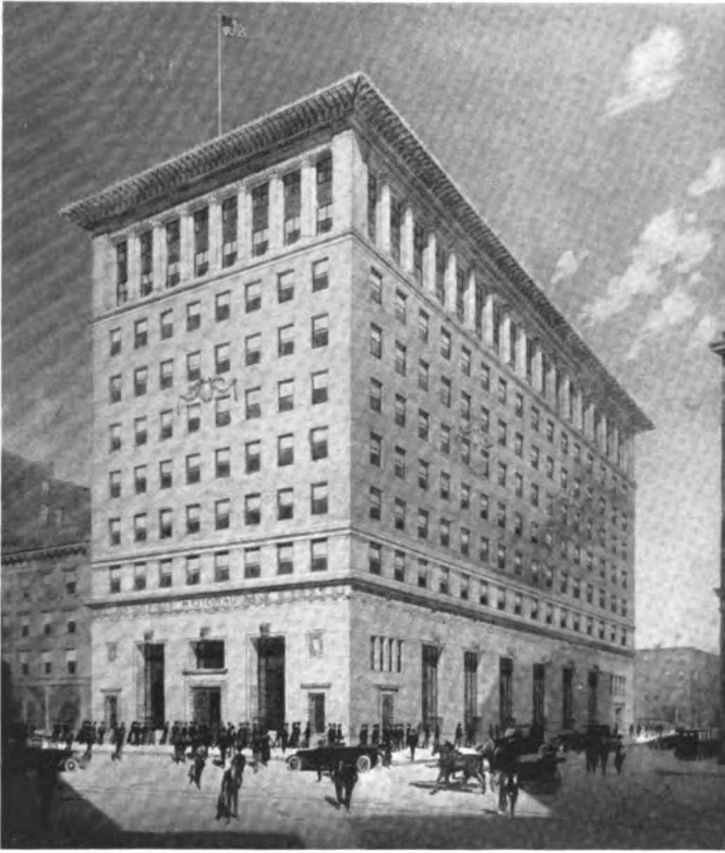
Externally an effort has been made to keep simple and dignified lines, consistent with the bank's business policy
