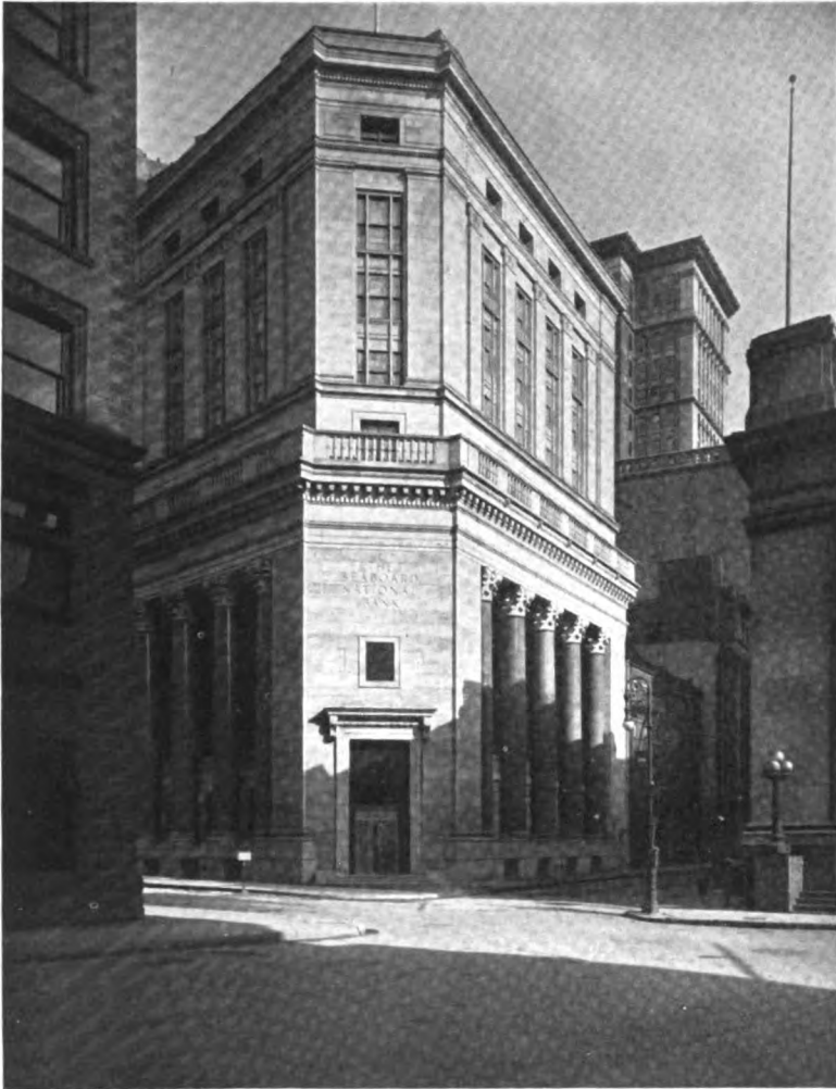
New home of the Seaboard National Bank, at the north-east corner of Broad and Beaver streets, erected from plans by Alfred C. Bossom, New York architect, which was chosen for first honors as best of the new buildings of down-town New York.
