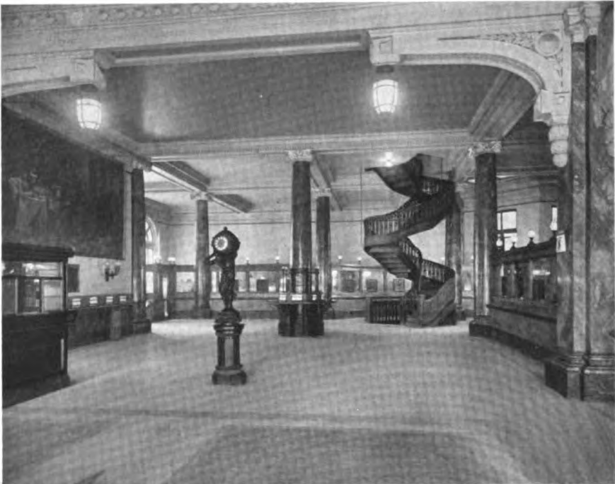
Main banking room, head office
