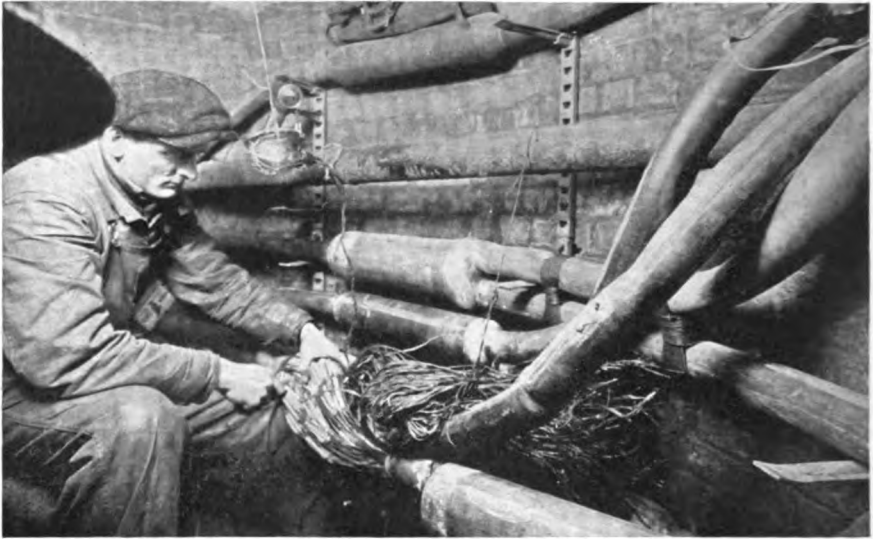
Splicing an underground cable
