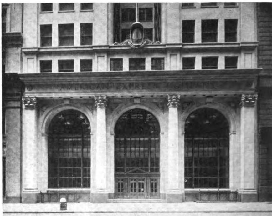
Facade of main entrance
