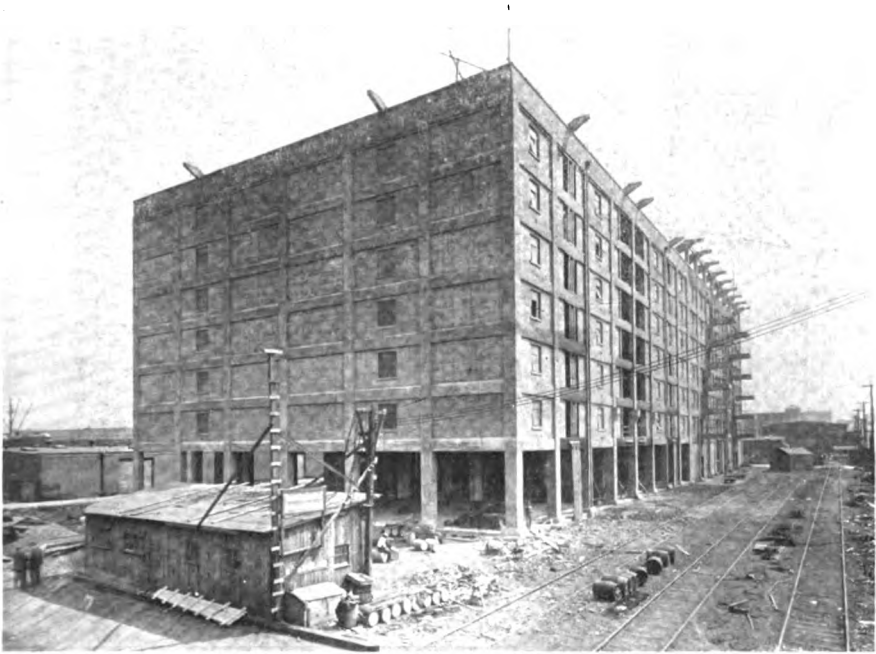
New warehouse unit under construction
