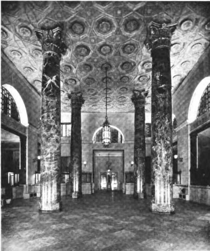
Main banking room of the new office of the New York Trust Company at 100 Broadway
