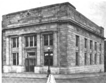
County National Bank of Lincolnton, N. C.
