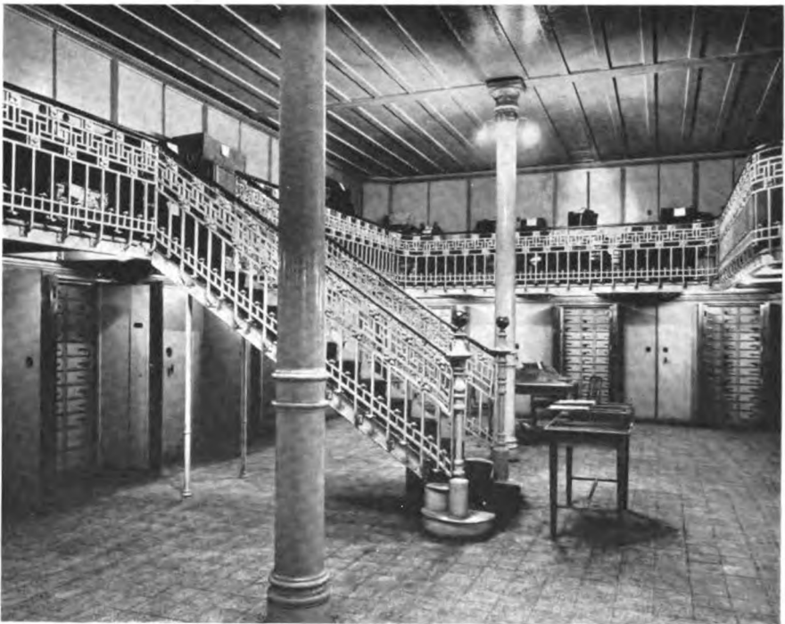
Safe Deposit Vaults at the Home Office
