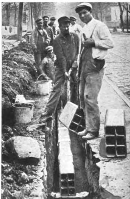
Subway construction, laying tiled ducts
