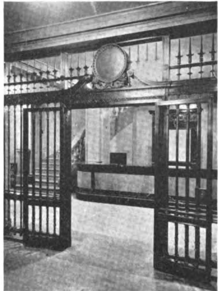
Grilled entrance to the safe deposit vaults
