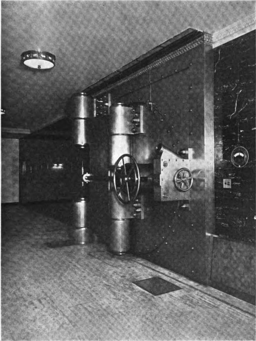
VIEW OF MASSIVE DOOR CLOSED
