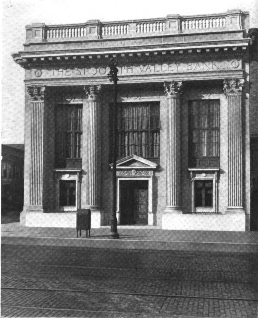
FULL FRONT VIEW OF THE EXTERIOR
