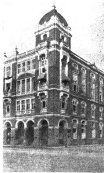
The Central Bank of India, Ltd., Hornby Road, Bombay
