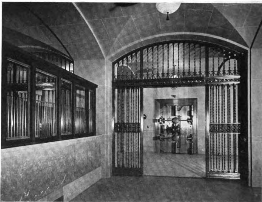
Entrance to the safe deposit vault
