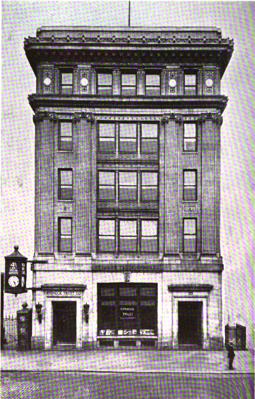
This entire Steneck Building was used by the Government during the war
