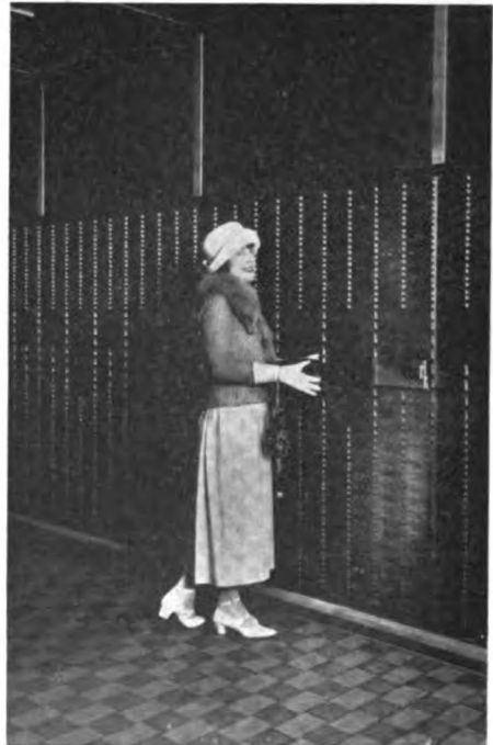
Section of safe deposit box installation
