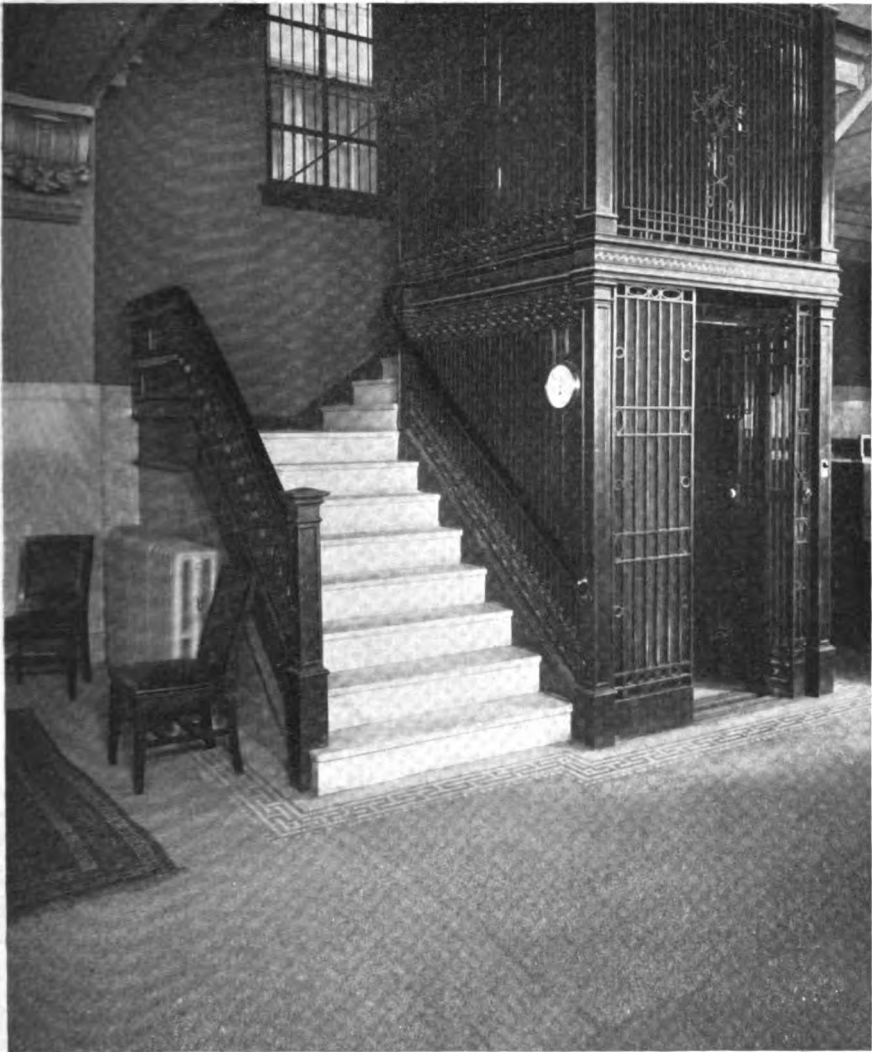
Self-Operating Elevator and Stairway Connecting Four Floors and Basement
