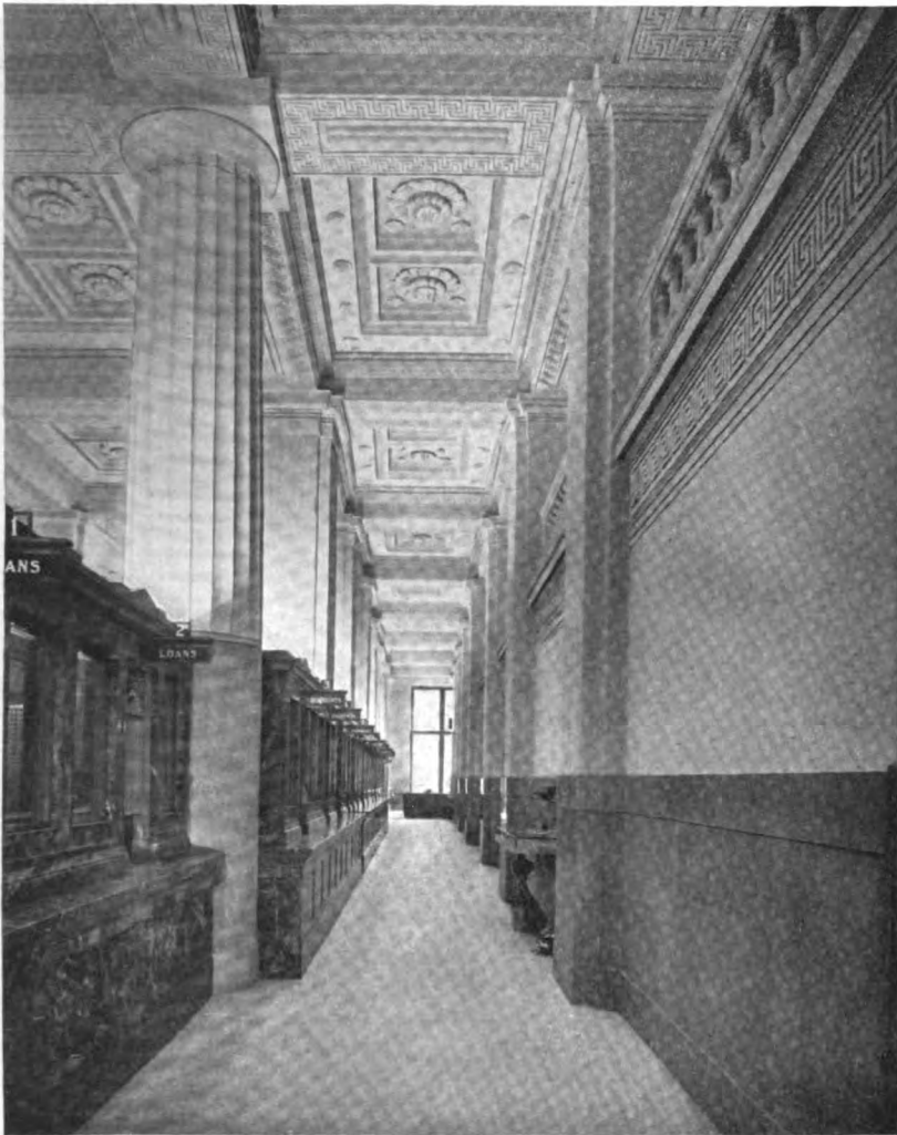
Vista of Banking Lobby Showing Indirect Lighting Effects
