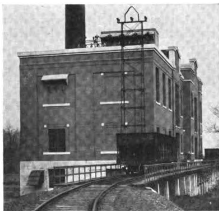
Williamsburgh Power Plant Penn Central Power and Transmission Co., Williamsburgh, Pa. This company is under Day & Zimmermann management
