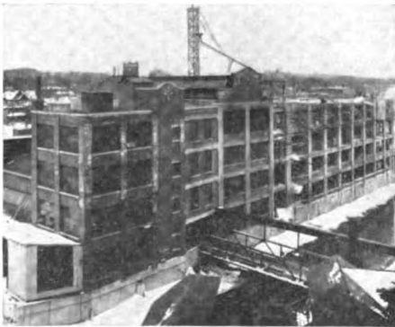
Plant for the New Process Gear Corporation Syracuse, N. Y.
