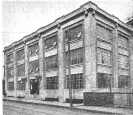
Offices of the Penn Central Light & Power Co., at Altoona, Pa. This company is under Day & Zimmermann management
