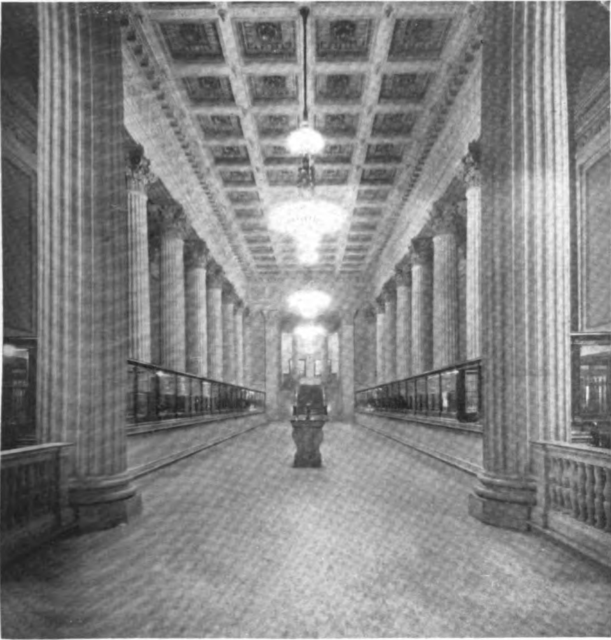
Main Banking Room. The Guardian Savings and Trust Company, Cleveland, Ohio
