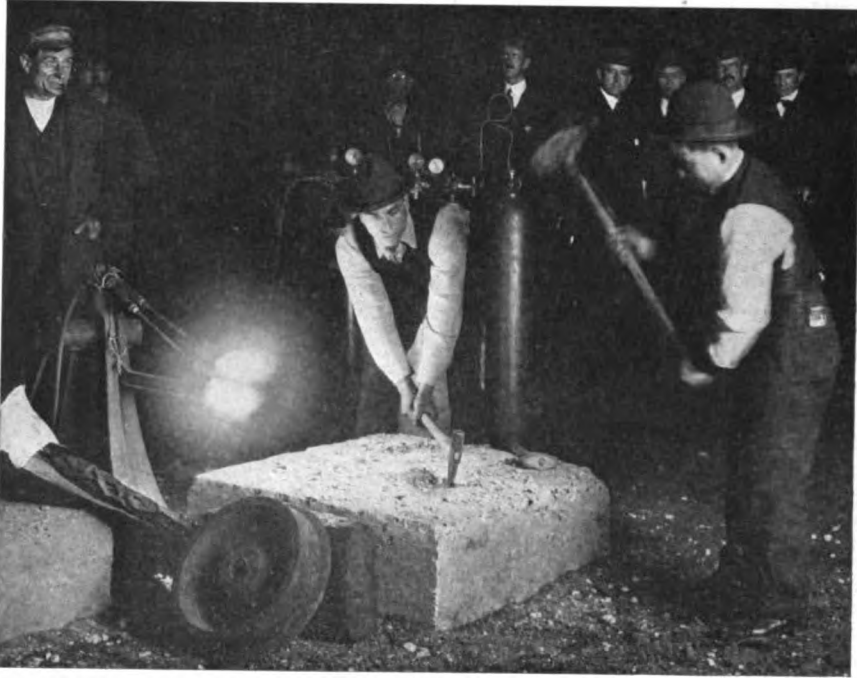
Attacking the heated concrete immediately after removing the torch
