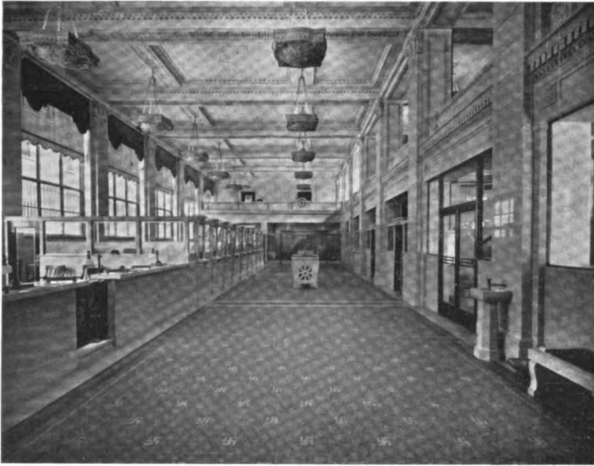
Interior, looking from Entrance, Old State National Bank, Evansville, Ind.
