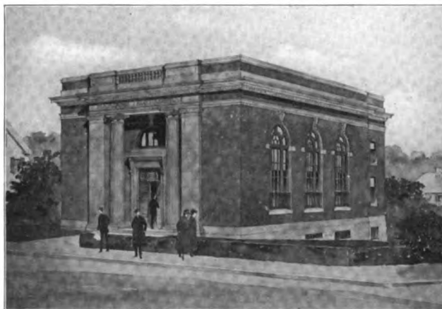
Proposed Building for the Rockland Trust Co., Rockland, Mass. Thomas M. James, Architect
