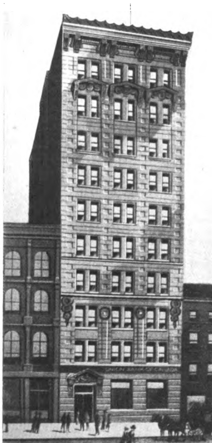
Montreal Branch, Union Bank of Canada
