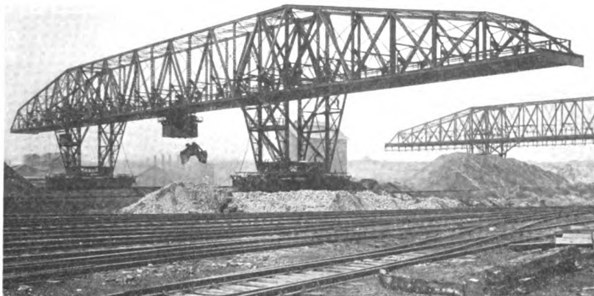
View of Traveling Cranes or "Ore Bridges" in Bethlehem Steel Company's storage yard
