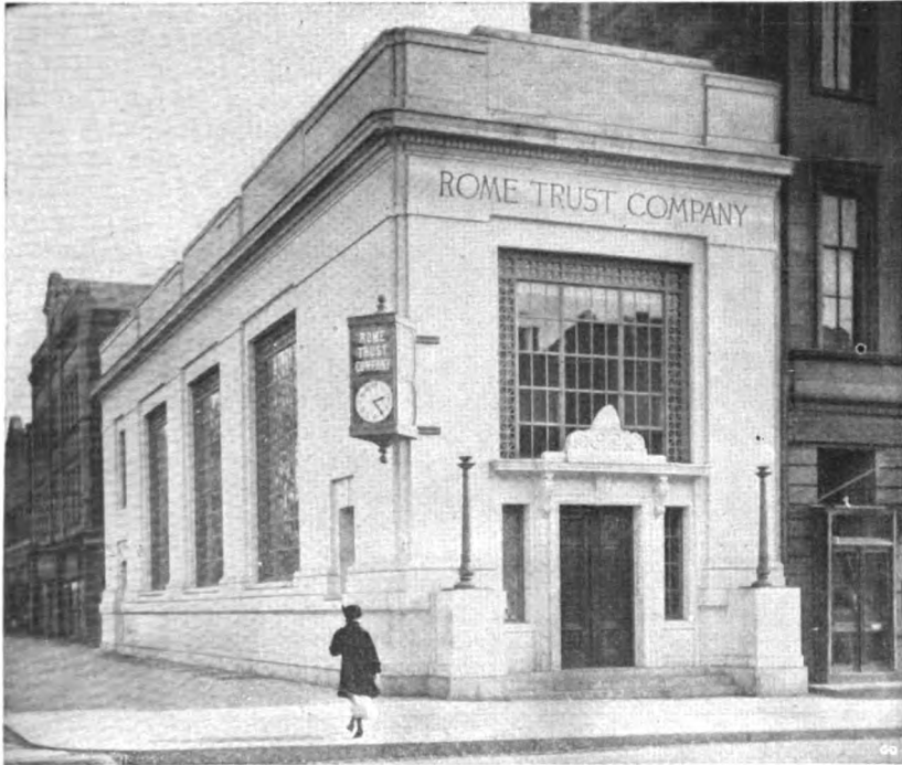
Indiana Limestone Banking Building of the Rome Trust Company, Rome, N. Y.
