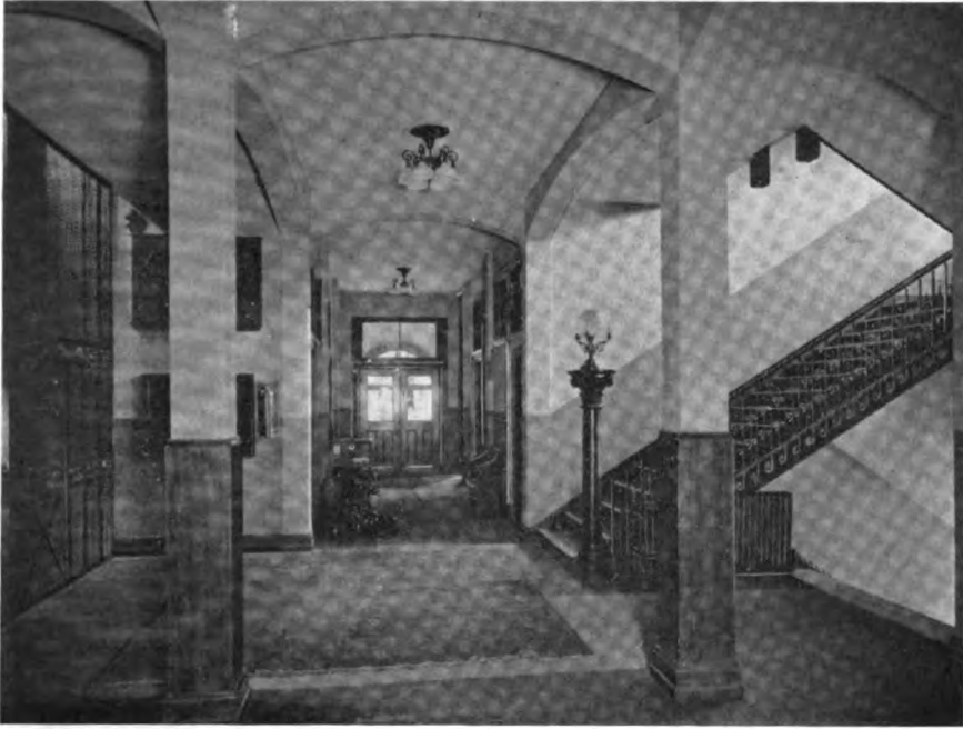
The Main Corridor on the First Floor
