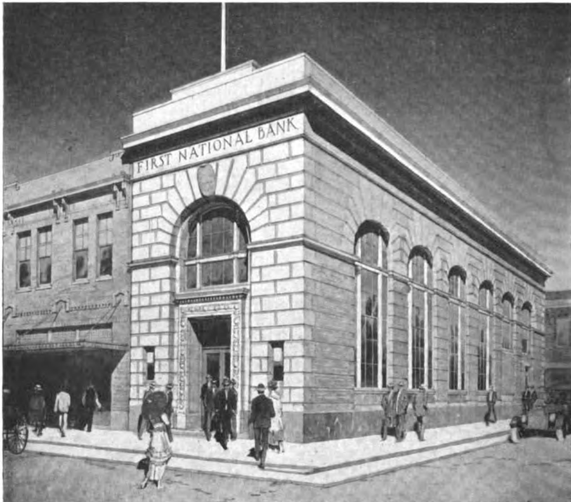
Distinctive individual Italian Renaissance bank building under construction by Hoggson Brothers, Builders, New York, Chicago and Atlanta, for the First National Bank of Bryan, Texas
