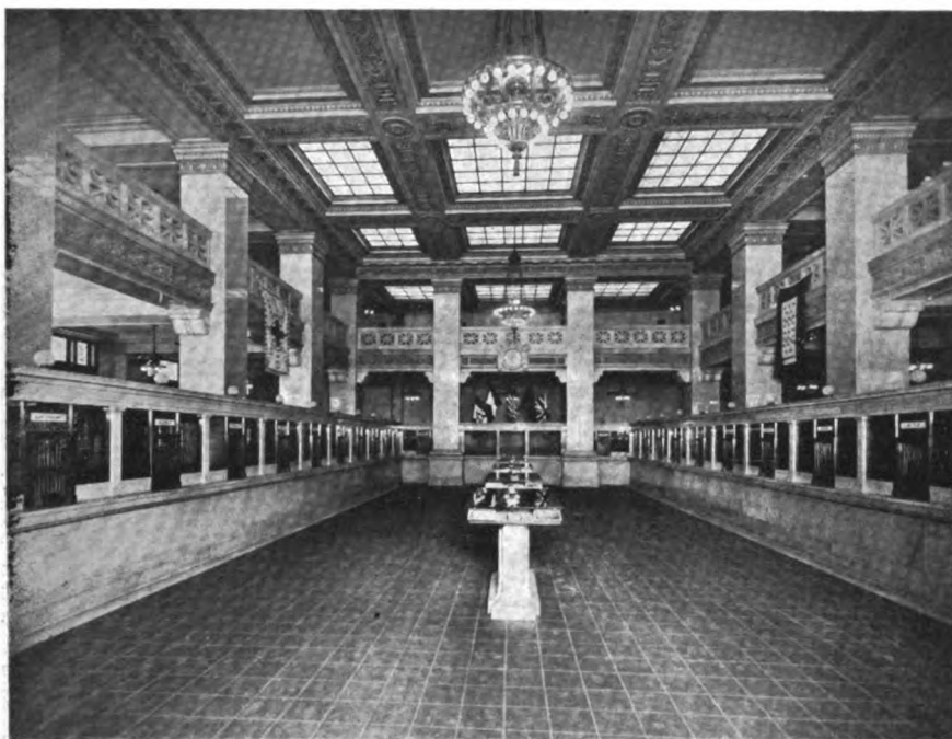
Main Banking Room and Public Lobby
