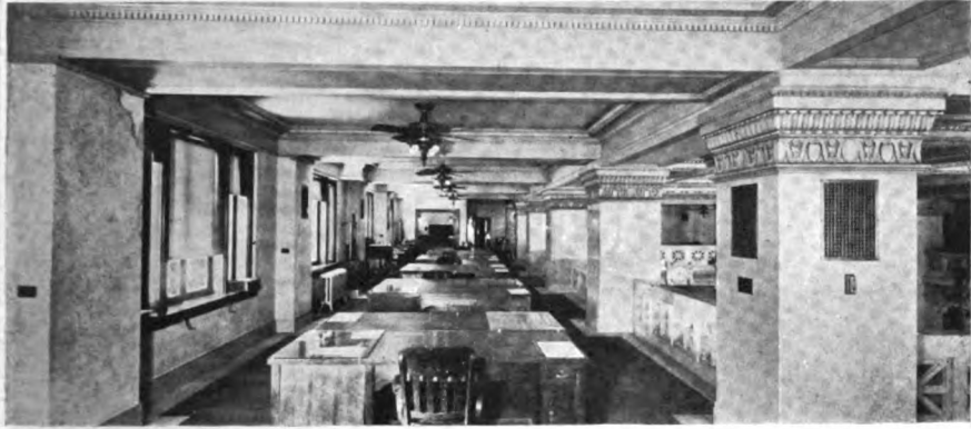
Mezzanine Floor Looking North
