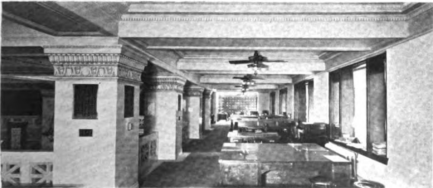
Mezzanine Floor Looking East
